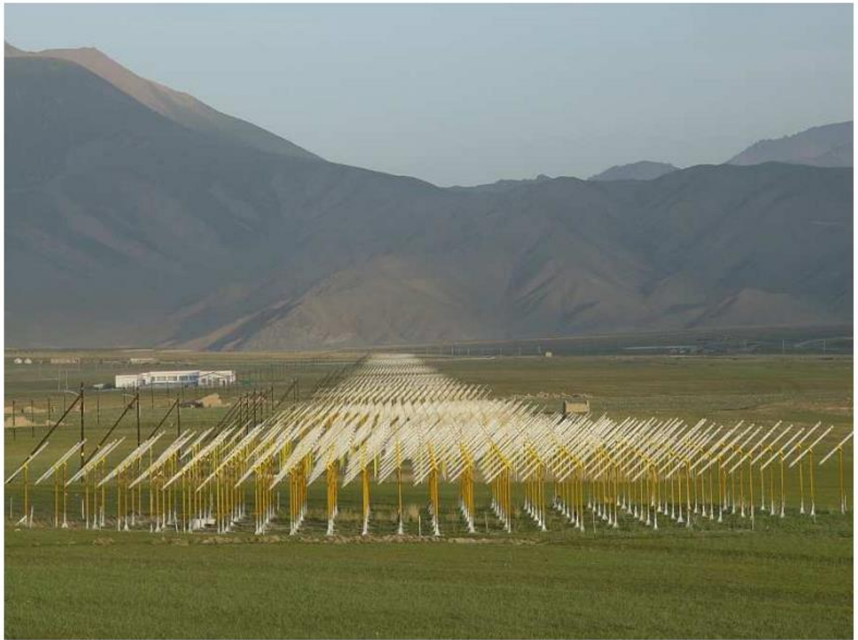
Fig. 3.— Photograph of the east-west baseline of the 21CMA, as seen from E17. The 'white house' to the left is the control center.
